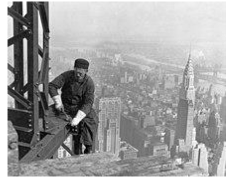
Construction on the Empire State Building was a symbol of U.S. economic growth after the First World War .
